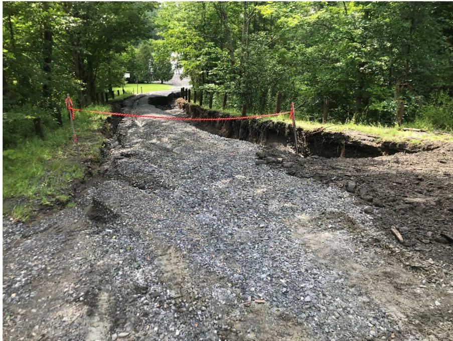
Figure 3. Storm damaged facilities – Gale Meadows Dam (top) suffered a significant washout as water overtopped the auxiliary spillway and eroded much of the large boulders. Rood Pond's (bottom) access road was washed out due to an undersized culvert under a town road. Debris was deposited on the boat ramp and in adjacent areas in the pond.
