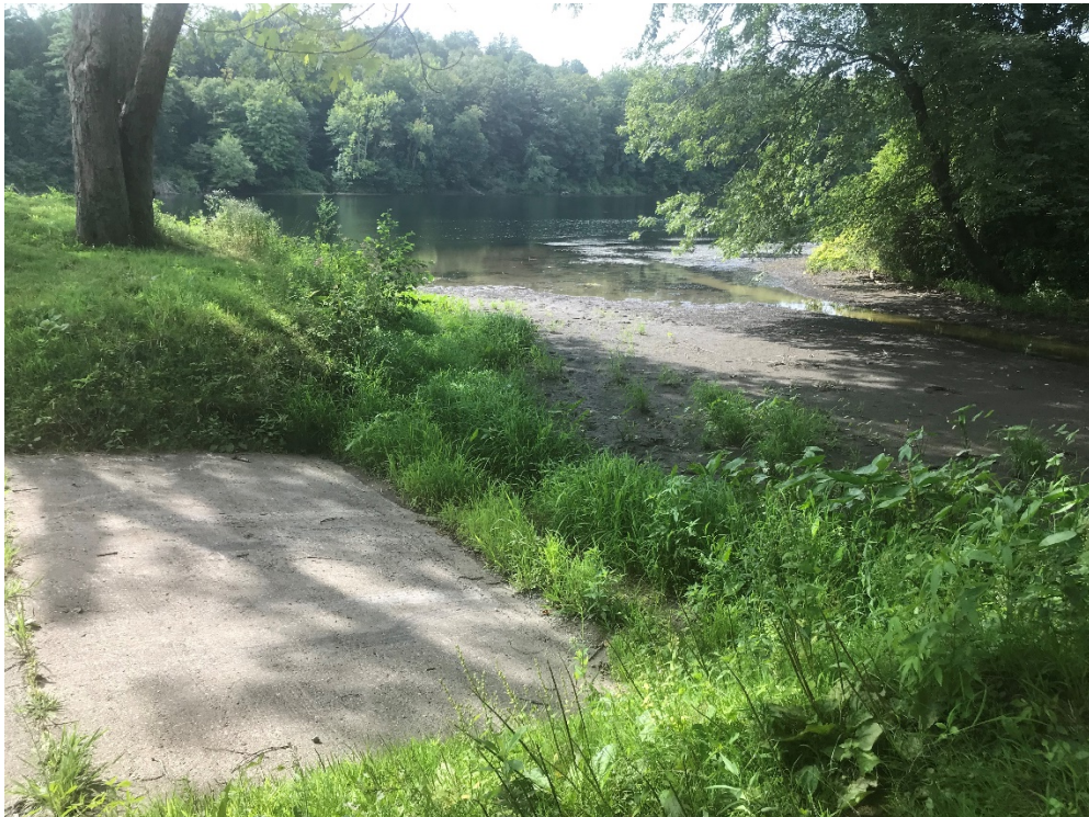
Figure 2. A new ramp (top image) was constructed this past summer at the Dummerston Access Area on the Connecticut River in Dummerston, VT. The old ramp (bottom image) was located in a small back water that had been completely filled with silt and was no longer usable.
