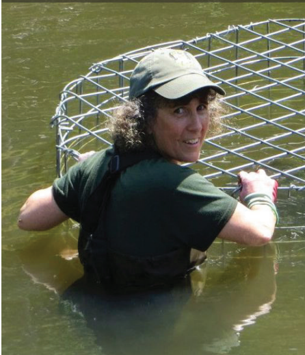
Mary Beth on the job installing a beaver exclusion fence.
