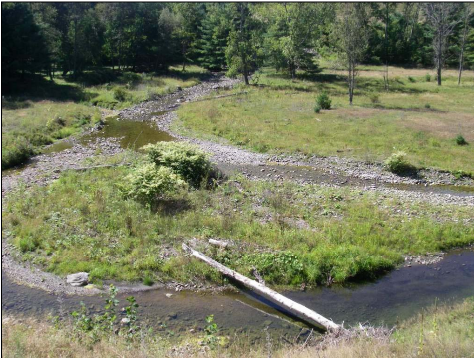
Figure 3. Downstream channel looking towards the culvert. The culvert is just out of view in the upper center of the photo.
