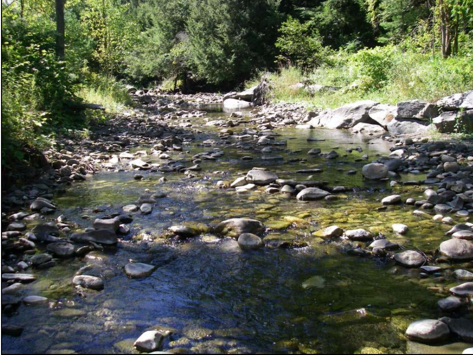
Figure 2. Upstream channel looking upstream from the culvert inlet.
