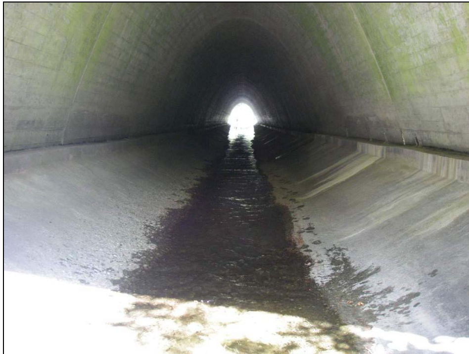
Figure 1. Interior of existing culvert from inlet looking downstream.
