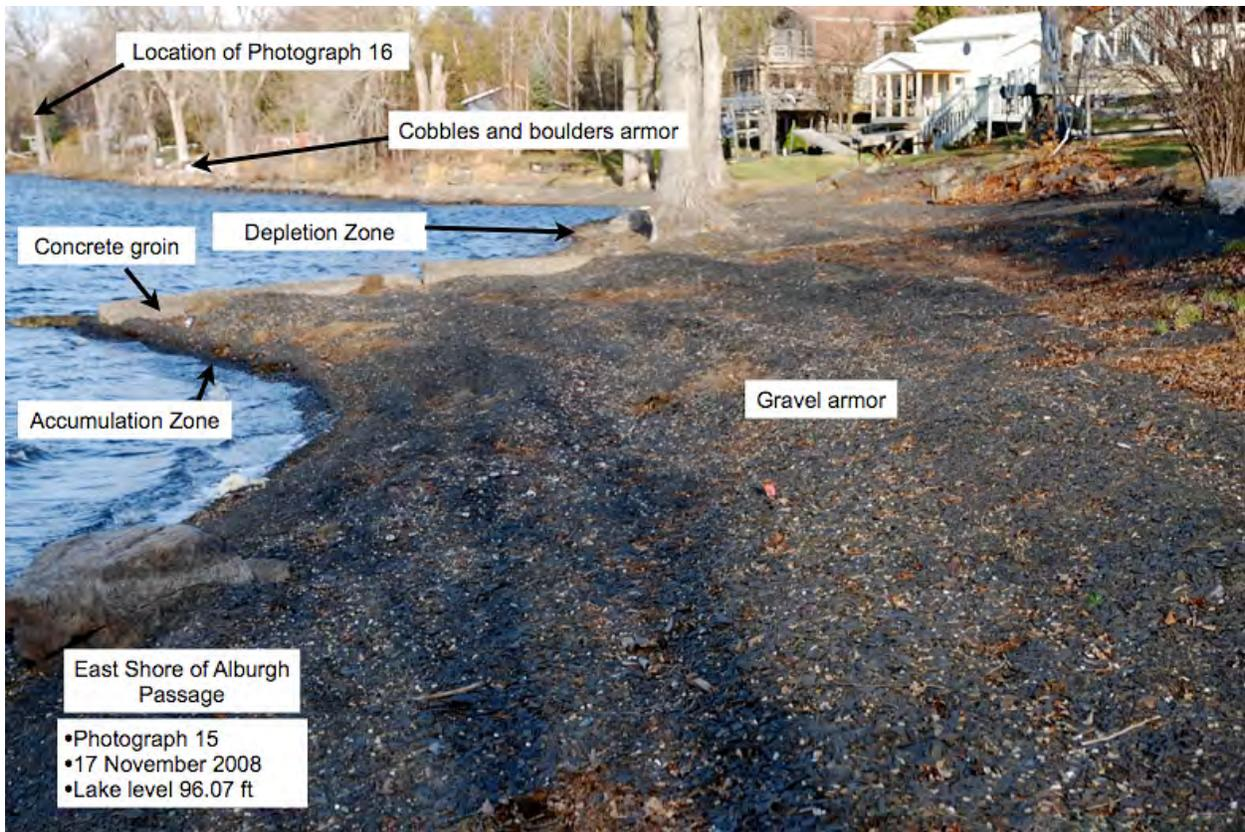
**Photograph 15** - Photograph 15 depicts the east shore of Alburgh Passage looking north. The groin, which is made of concrete in addition to boulders, traps gravel. Further north more cobbles and less gravel are evident. The mean weight of eight cobbles selected from the beach north of the groin was 4.8 pounds.
