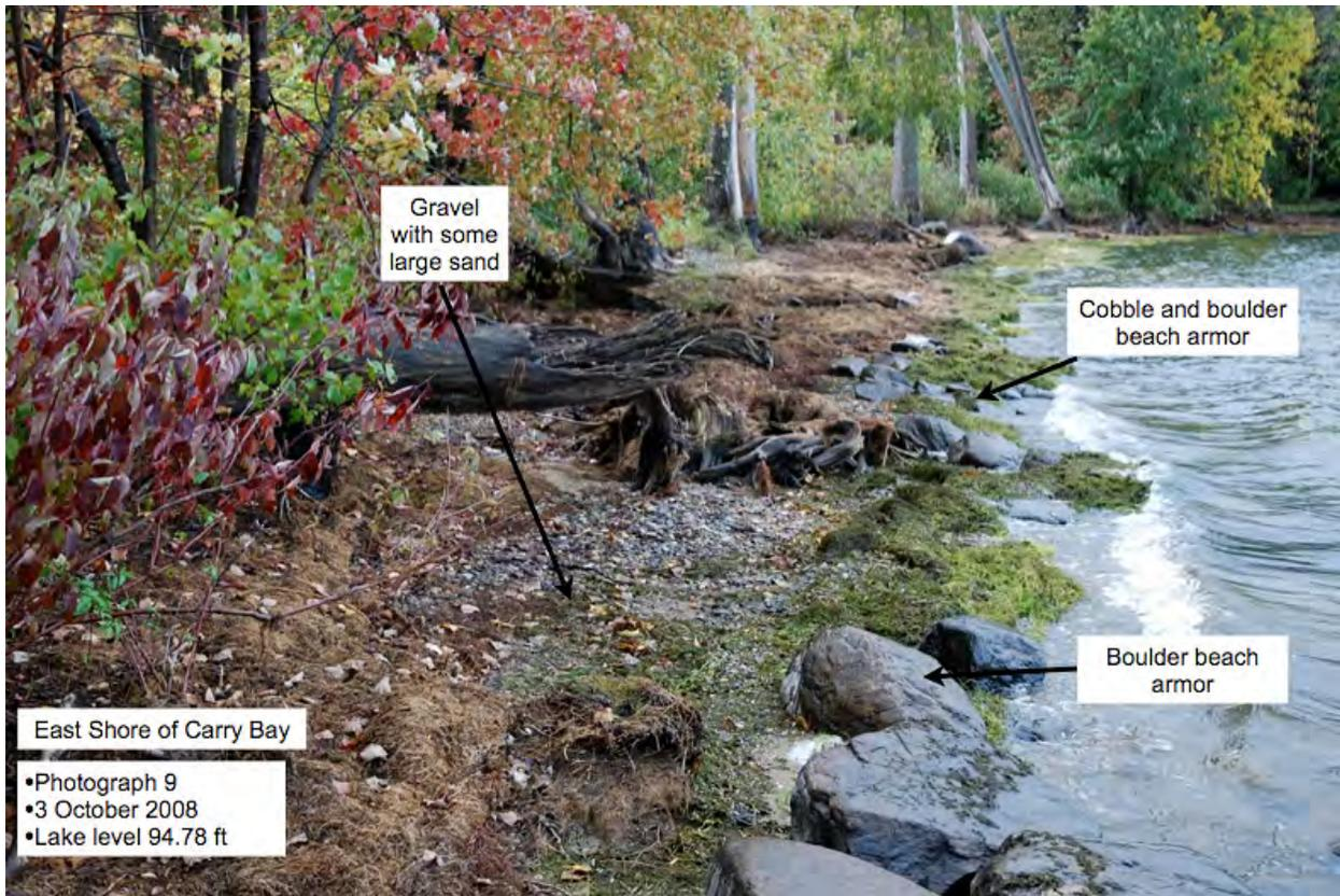
**Photograph 9** - Photograph 9, taken on October 3, 2008, also depicts boulders along the edge of water, but this section of beach is not bordered by a bedrock bank as seen in Photograph 8. Sections of this beach have deposits of sand, which is rare for beaches in the study area. The low elevation of the backshore appears to flood at higher lake levels.
