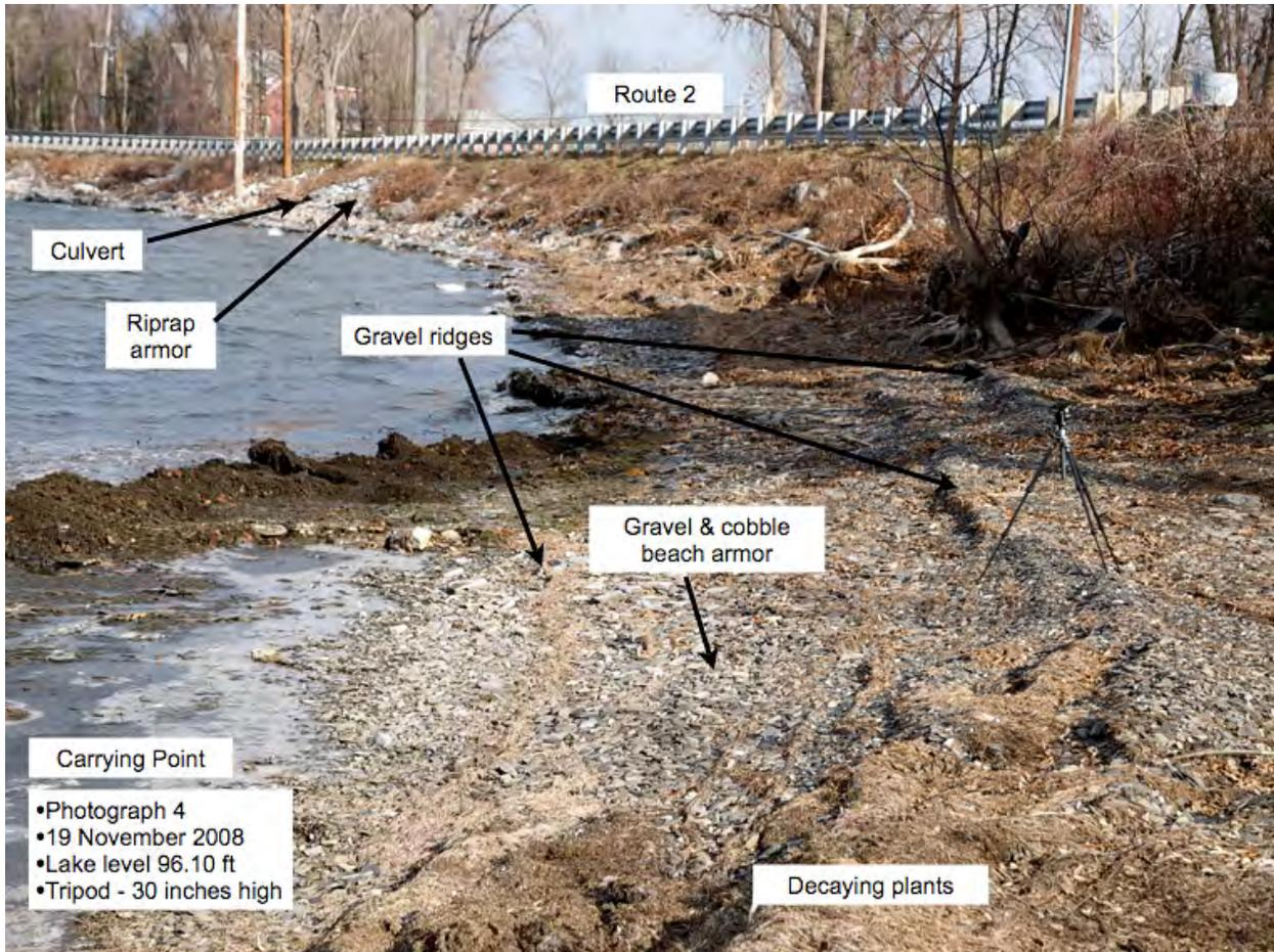
**Photograph 4** - This picture was taken looking north close to the “Carrying Point.” This area has been greatly modified and a steep riprap bank extends along the shore. A culvert provides very little exchange of water between Carry Bay and the Inland Sea. Gravel ridges appear along the shore where wave action piled gravel size rocks in rows parallel with the edge of water. A large amount of decaying plants were along the shore.
