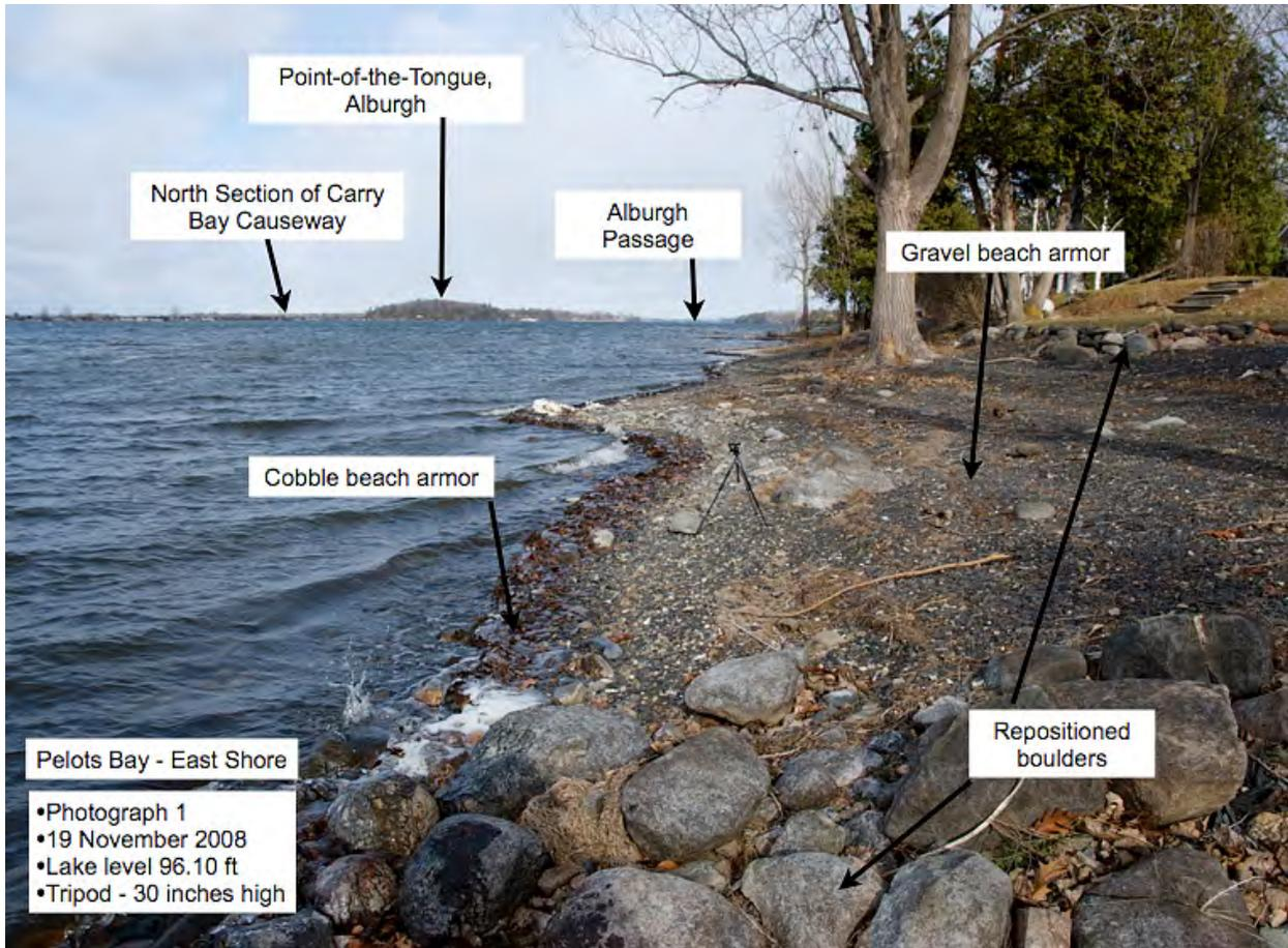
**Photograph 1** - This picture was taken looking north along the west shore of Pelots Bay and south of Savage Point. Boulders were moved and grouped together to construct walls and groins. The beach slope extends landward and ends at the base of the stairs seen in the upper right where permanent vegetation begins. Cobbles dominant from the edge of water and offshore (foreshore) while gravel are more plentiful landward (backshore).
