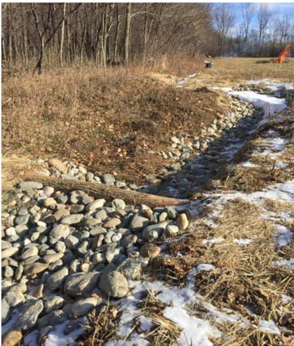
Log-based check dams help to minimize erosion and sediment transport in drainage gullies and improve water quality.
