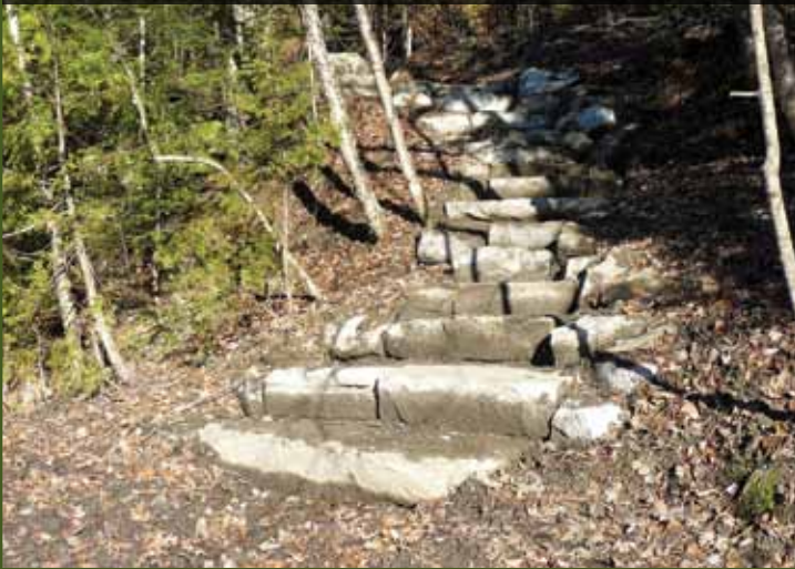
Granite steps constructed using "wall stone" donated by Rock of Ages prevent erosion and will provide access for viewing steelhead trout jumping at Willoughby Falls for many generations. Photo: Paul Hamelin - VFWD
